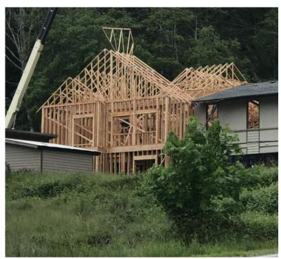
The old roof is being removed and the new trusses are going up.
